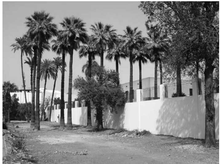
The completed wall from outside
