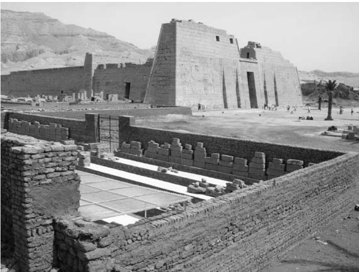
The blockyard with roofing
