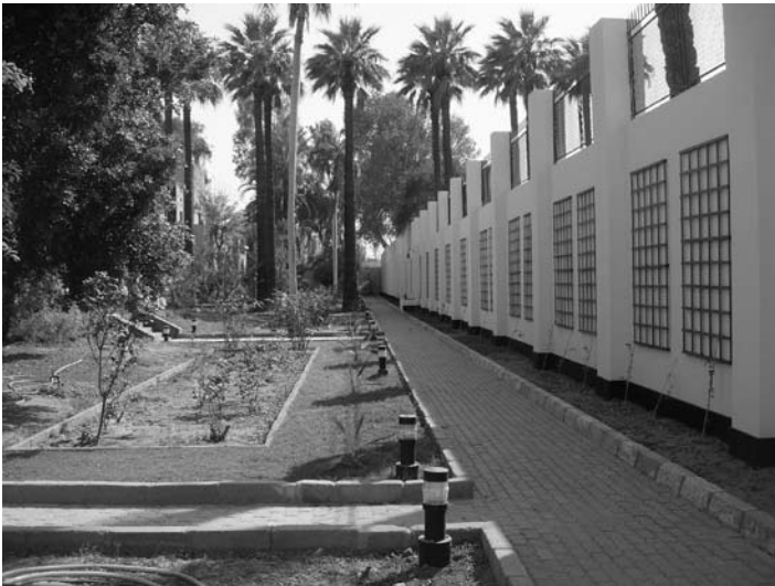
The completed wall from inside
