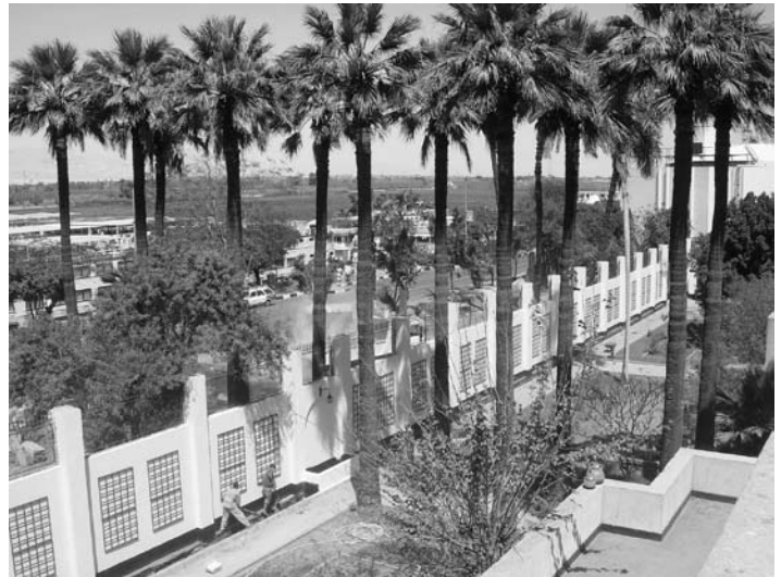
The completed wall from above
